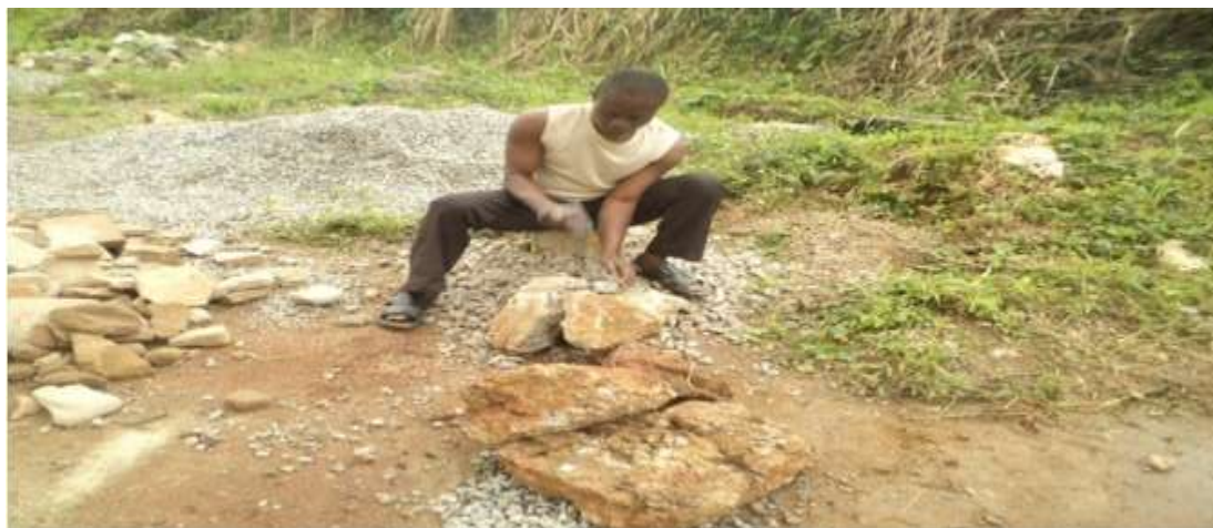
Plate 2.1c: Showing the process of breaking the demolished concrete
