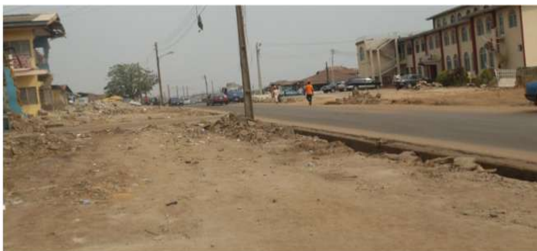
Plate 2.1a: Arakale Street Undergoing Building Demolishing Due to Road Dualization.
