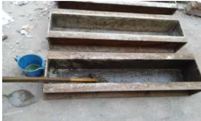
Figure 4. Formwork preparation for beam specimen.
