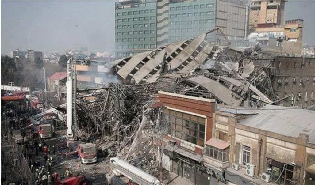
Fig 3. Plasco Building demolition [4]
