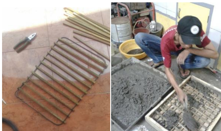
Fig 3. The process of making water gates from panels with reinforcement from bamboo
