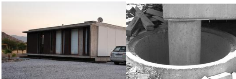
Figure 2. Housing with seismic isolation system PPP [4].
