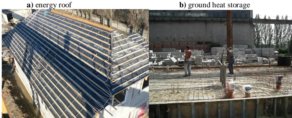
Figure 4: Solar energy roof and ground heat storage built into and under the foundation slab of a type panel house IDA I. (photo archive: Kalús, D.) [7, 8, 9]
