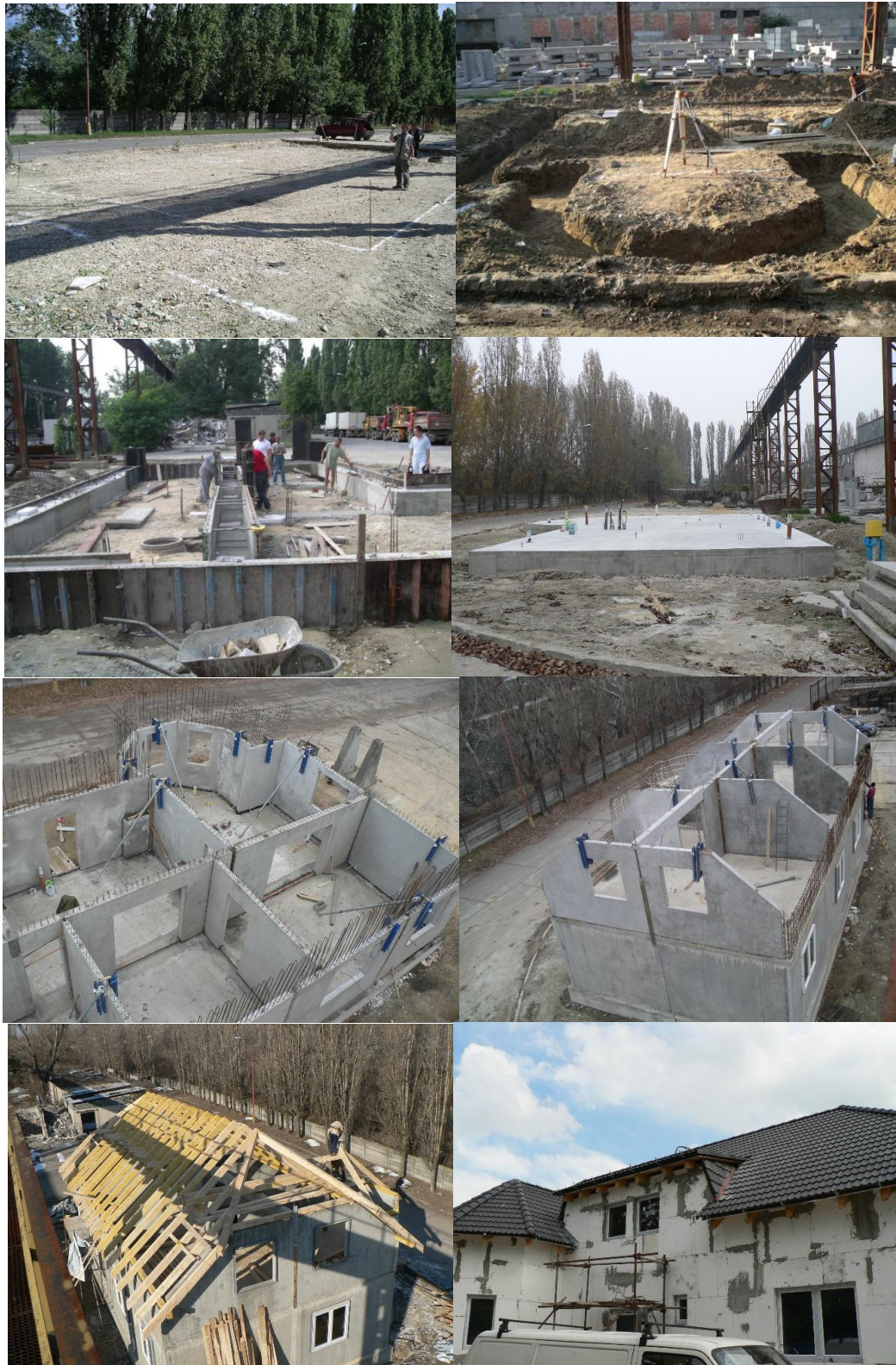
Figure 3: Photographs from the assembly of type panel house IDA I. (photo archive: Kalús, D.) [7, 8, 9]
