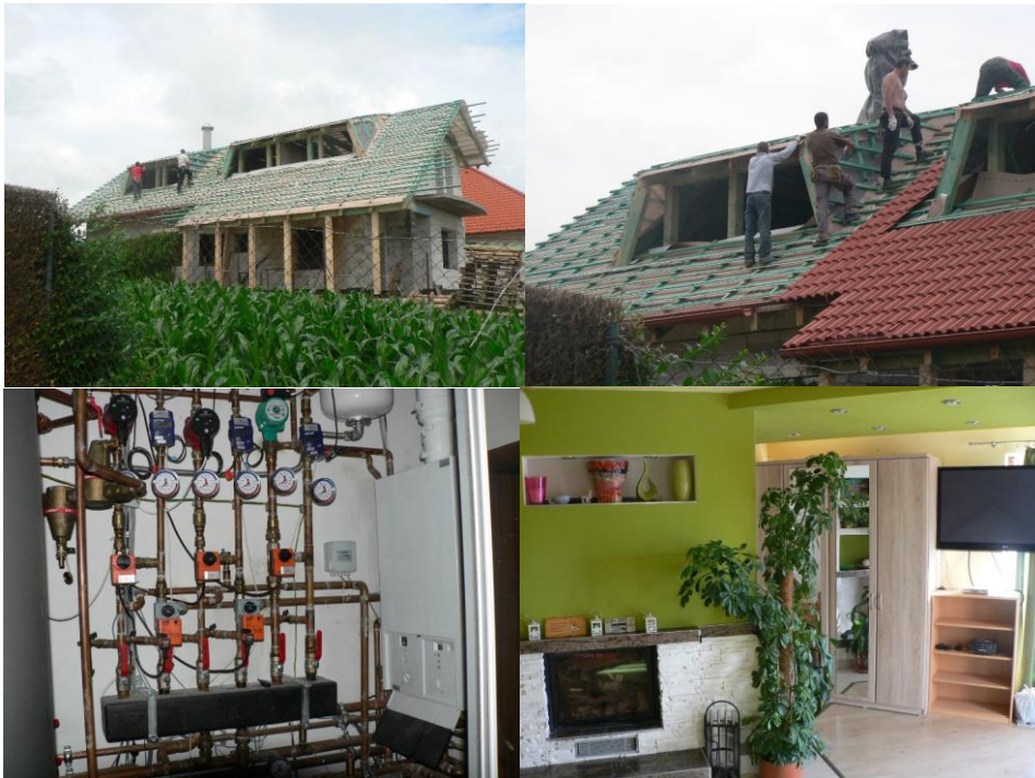
Figure 3: Energy roof consisting of plastic pipes under roof tiles, a low-temperature gas boiler and a fireplace with a hot water heat exchanger (Photo archive: Kalús) [10, 13]
