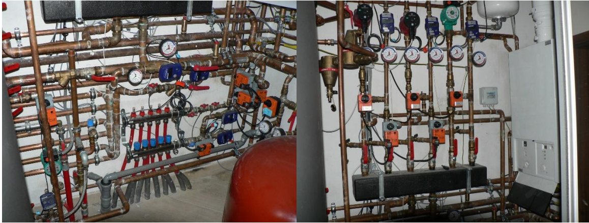
Figure 10: A view of the connection of energy systems in the experimental house EB2020 (Photo archive: Kalús) [10, 13]
