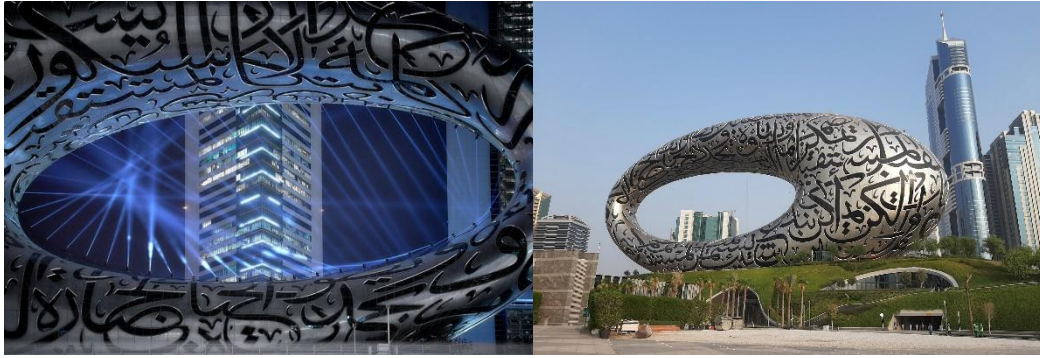
Figure 3. Stainless-steel-clad glass fibre reinforced plastic (GFRP) form the building's landmark facade.
