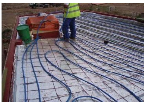
Figure 4: Absorber from a plastic pipe placed on the roof structure, the top layer of the structure will be a board with waterproofing, Spain [22]
