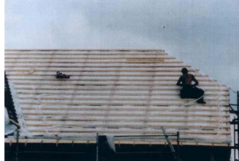
Figure 3: Plastic placed on the roof structure, the top layer will be roof tiles. Left: Slovakia, right: Luxembourg [20], [21]
