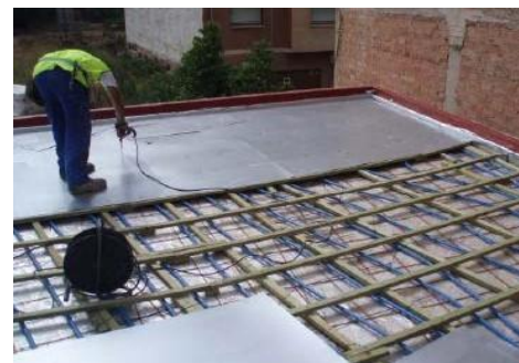
Figure 4: Absorber from a plastic pipe placed on the roof structure, the top layer of the structure will be a board with waterproofing, Spain [22]
