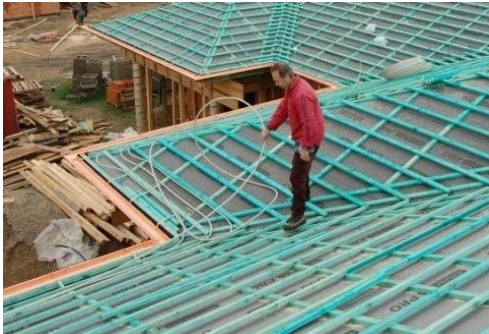
Figure 3: Plastic placed on the roof structure, the top layer will be roof tiles. Left: Slovakia, right: Luxembourg [20], [21]
