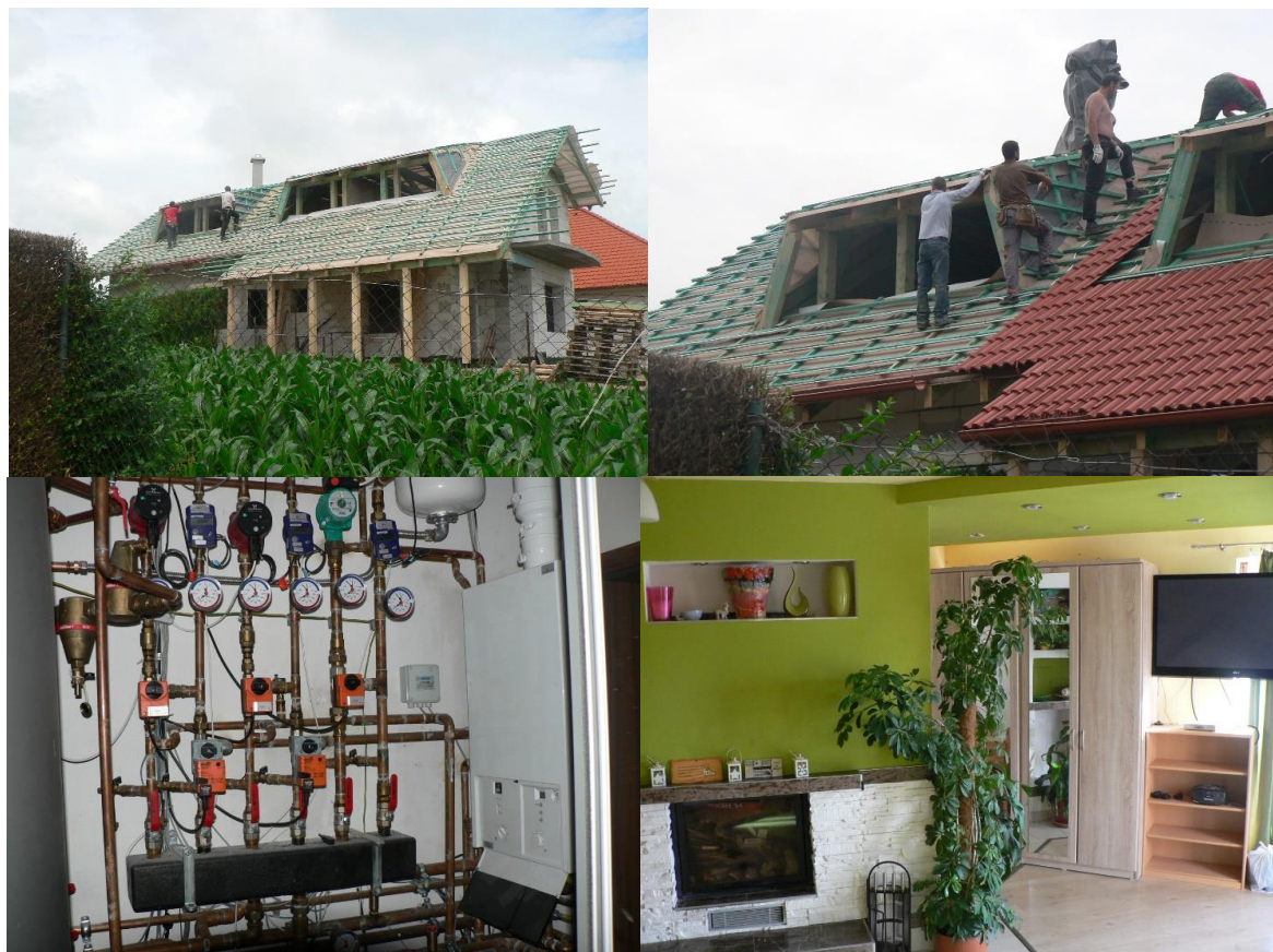
Figure 8: Energy roof consisting of plastic pipes under roof tiles, a low-temperature gas boiler and a fireplace with a hot water heat exchanger (Photo archive: Kalús) [10, 13]
