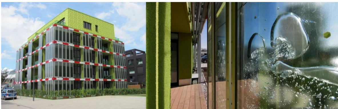
Figure 2b. Germany’s extraordinary “algae house” or BIQ building in Wilhelmsburg, Hamburg incorporates microalgae into its design [53]. One side of the green-hued tower’s transparent surface contains growing algae that controls light entering the building and provides shade when needed.
