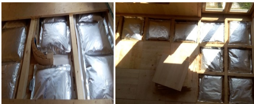
Figure7: Macro-encapsulated PCM [26]
