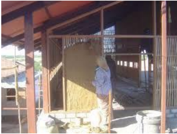
Image 3. Wall construction Khamir- Kutch Infill of wattle and Daub panel by local community in steel framework
