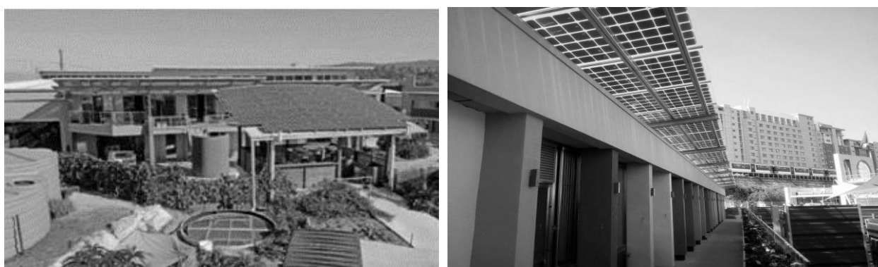
Figure (4) Solar Panel Combined with cantilever structure
