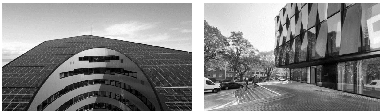
Figure (7) solar collector combined with façade
