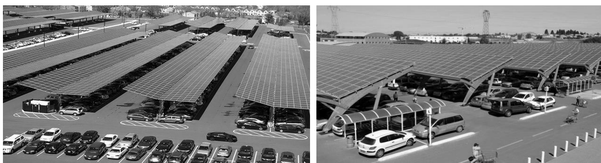
Figure (5) Solar Panel Combined with Parking Canopy
