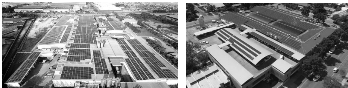
Figure (4) Solar Panel Combined with the roof
