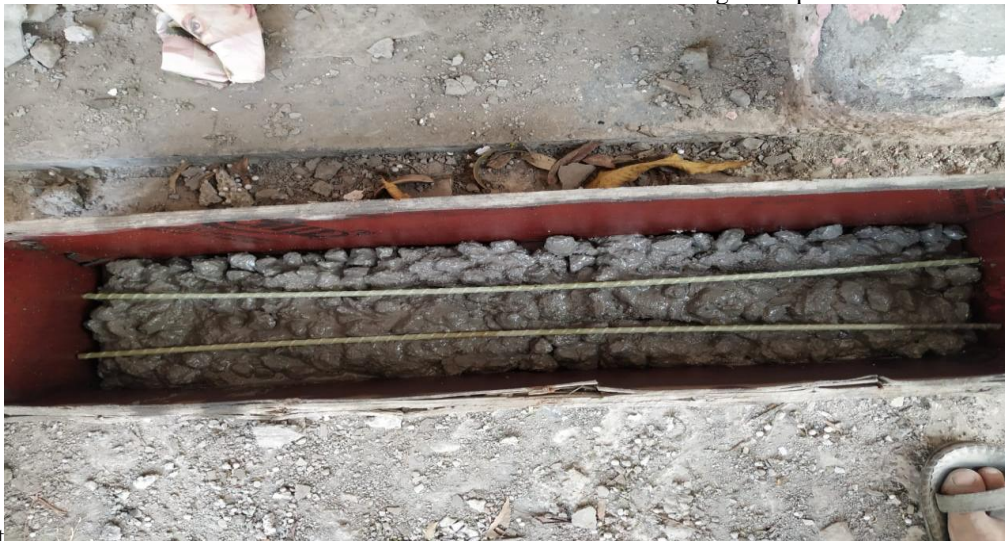
Casting of beam with FRP rebar in it
