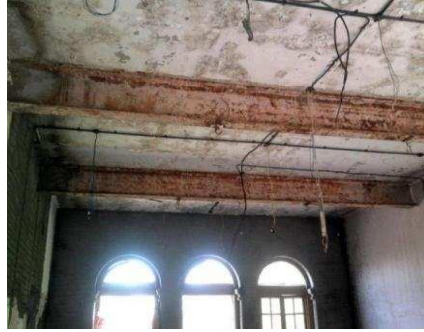
Figure 14 Roof leakage [1]
