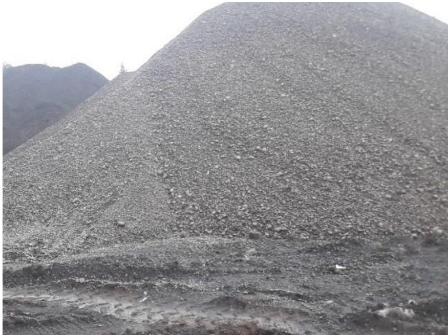
Figure 8: Good handling of sand and coarse aggregate on project site
