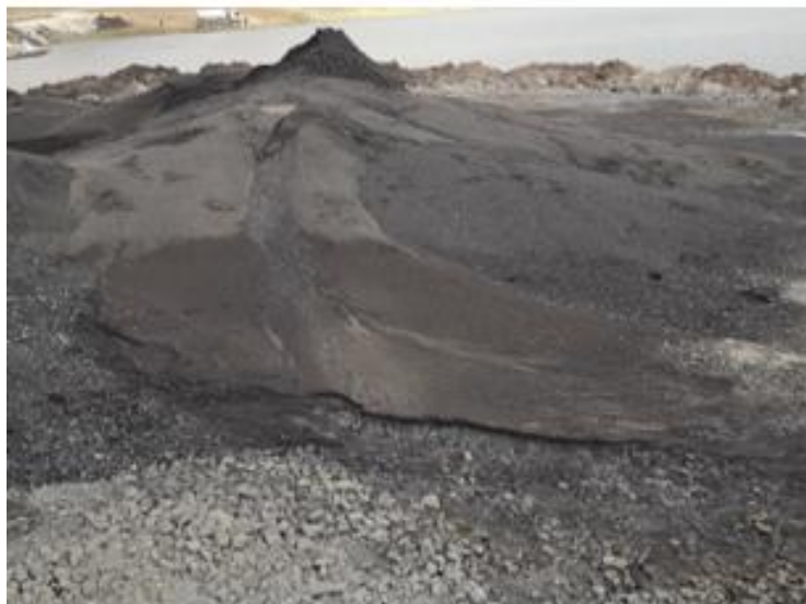
Figure 5: Improper Handling of Sand onsite
