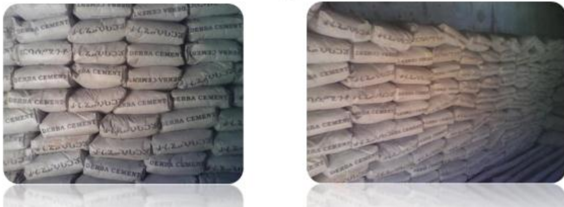
Figure 10: Recommended ways of storing cement on construction site
