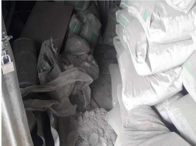
Figure 9: Wastage of cement due to poor handling, Lack of control & poor storage
