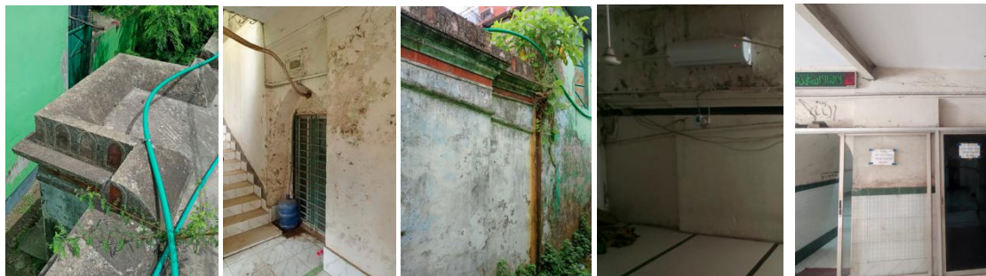
Fig.05 Exterior Parts of Yusufganj Mosque, Photos by, 1 st Author
