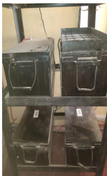
Figure 2: Battery Bank.
