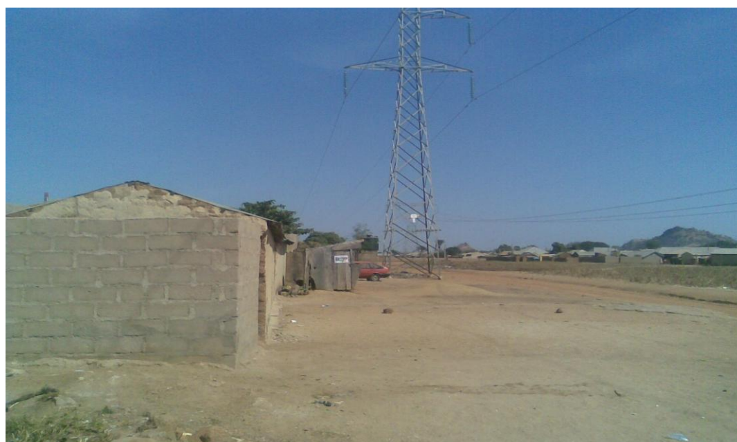
Plate 2 Encroachment In To High Tension Grid Line
