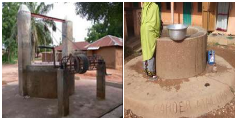
Photo assembling1: Large wells in Bagri (the one on the left is covered and quipped with a winch; the one on the right allows human force for water extraction and has no door)
