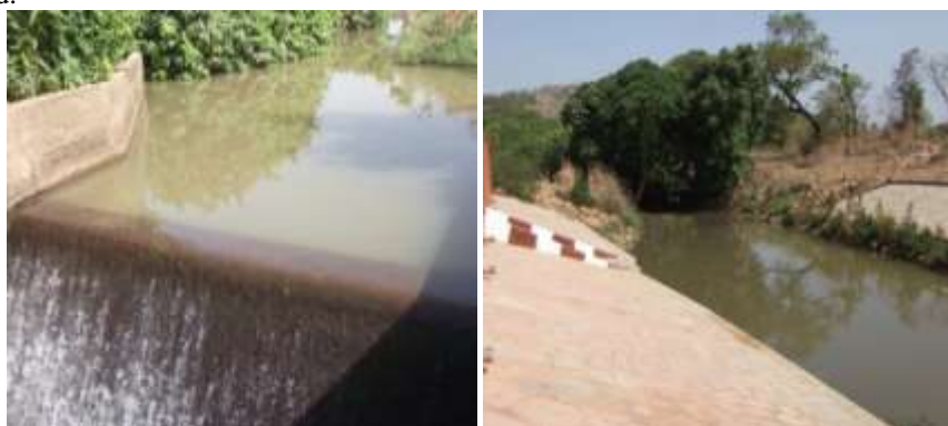
Photo assembling5: Spillway of the SONEBwater detention in Ouroubona
