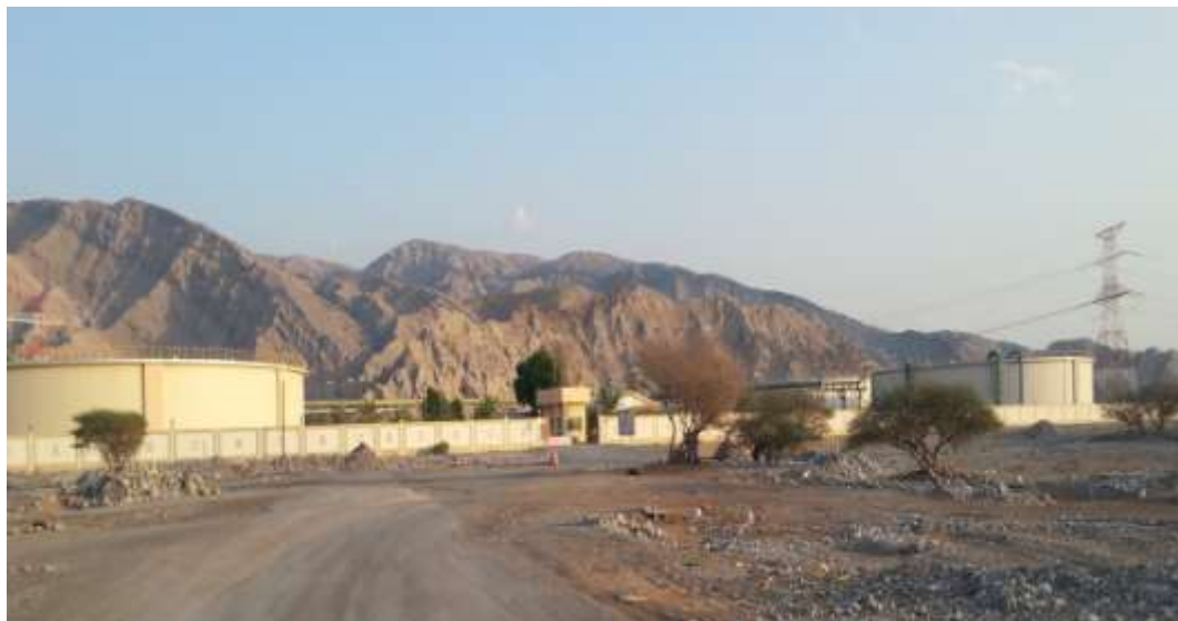
Photo 1. General view of storage tanks of Al Burayrat Reverse Osmosis (RO) Desalination plant in Wadi Al Bih area, Emirate of Ras Al Khaimah, United Arab Emirates.
