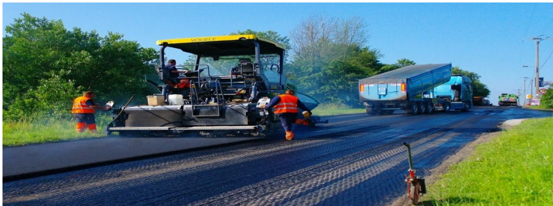
Plate 1: Typical Road Construction Works for Rural Infrastructural Development
