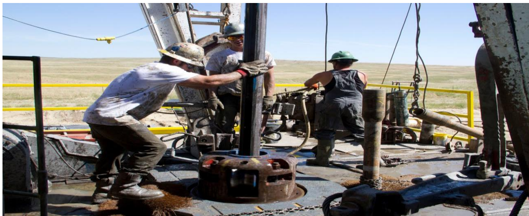
Plate 2: On-Going Geotechnical Works for Rural Infrastructural Development
