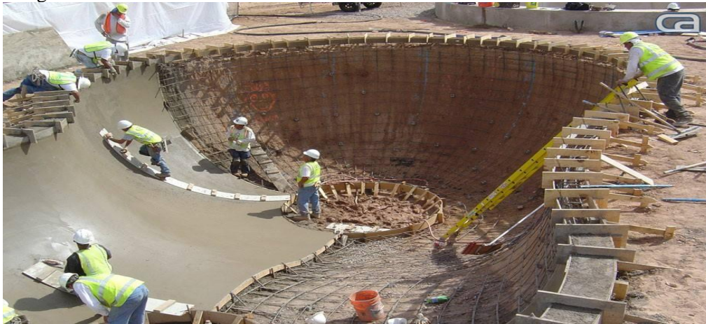
Plate 1: Effective Site coordination with efficient man-power in Lagos State
