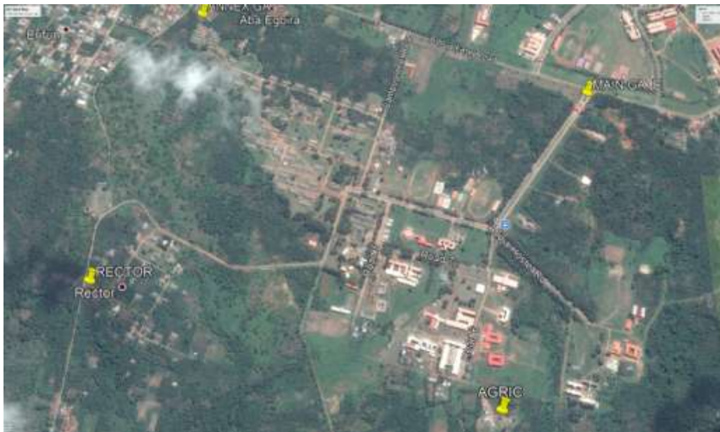
Fig.2: AN IMAGERY OF PART OF FEDERAL POLYTECHNICS, ADO-EKITI.
