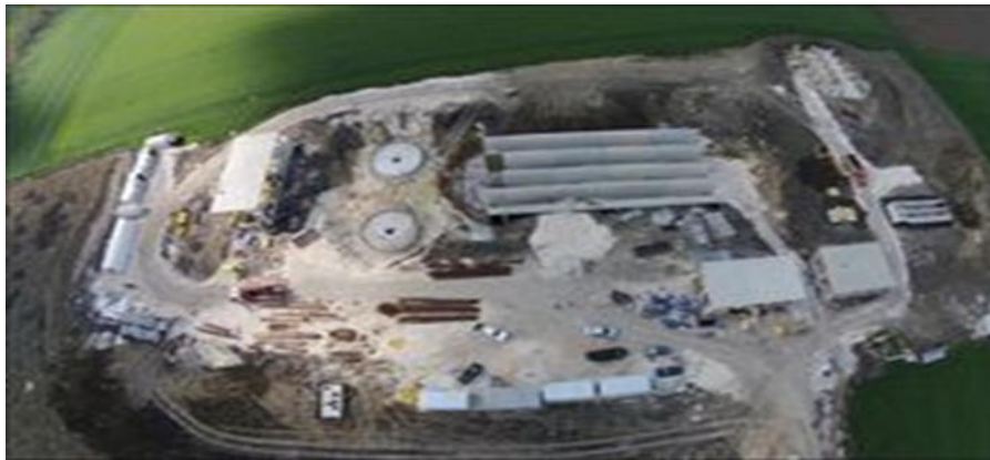
Figure 7. Pınarhisar Municipality waste water treatment plant [6]
