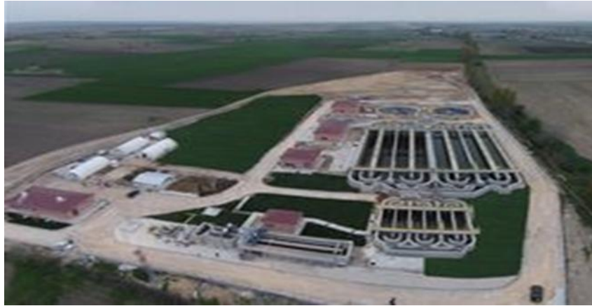
Figure 4. Kırklareli Municipality domestic wastewater treatment plant [6]
