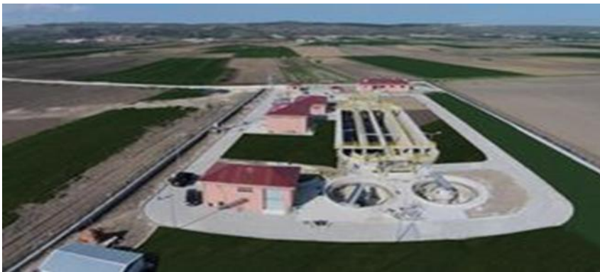
Figure 5. Vize Municipality domestic wastewater treatment plant [6]
