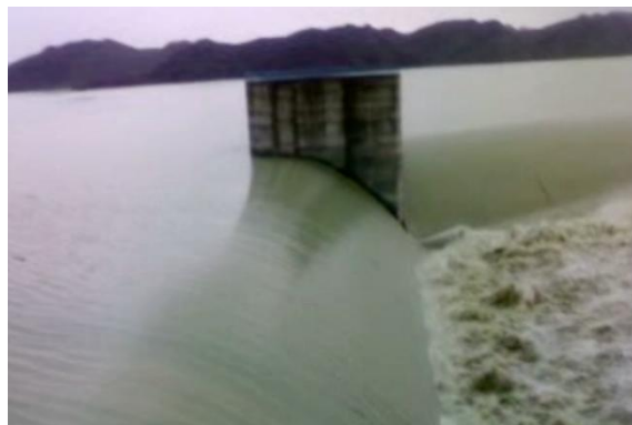
Figure 2: Spillway of the Pishin Dam with bankfull flow during flash flood in the stem of Sarbaz River 2020
