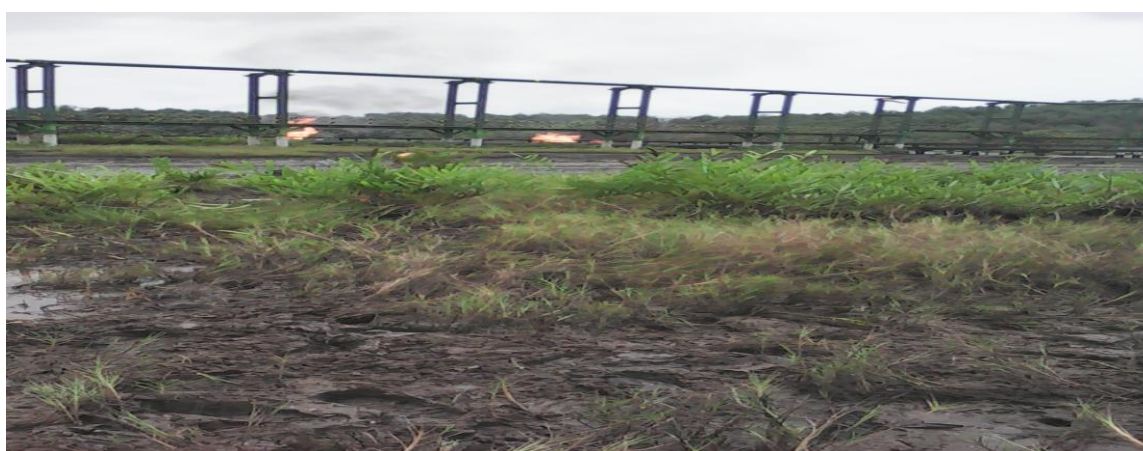
Study location showing Flare stack and open flaring
