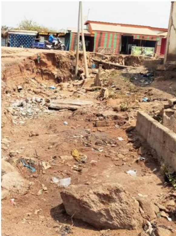
Photo 1: Road completely eroded by rainwater in the Karijourassokroneighbourhood (Shot: Bakary Nambahigué Mathieu, 2021)
