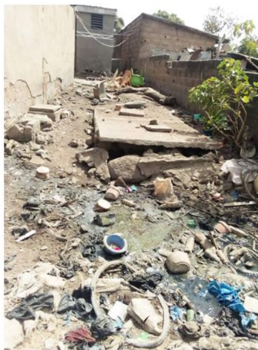
Photo 6: An open septic tank with black water flowing in a concession in the Djimisso district (Shot: Bakary Nambahigué Mathieu, 2021)
