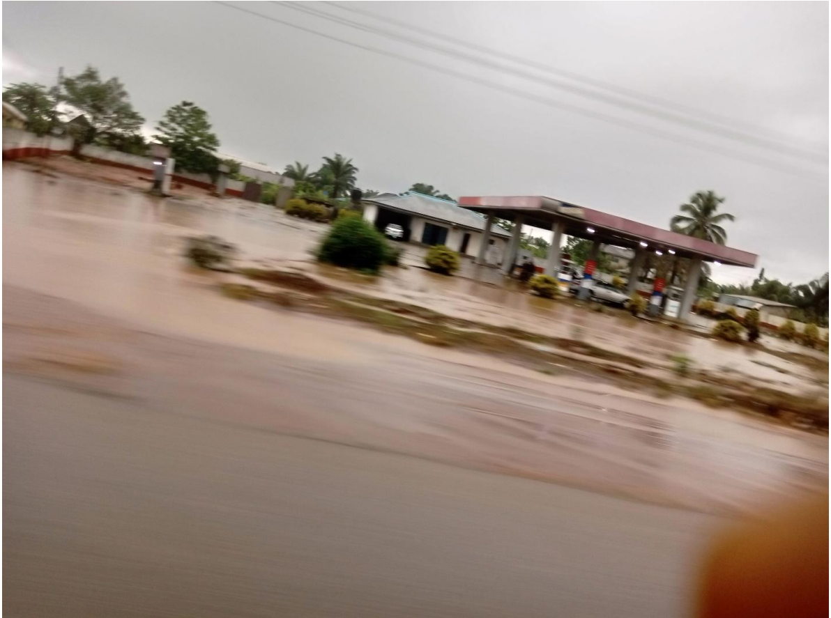
Plate 3: Petrol filling station covered by flood
