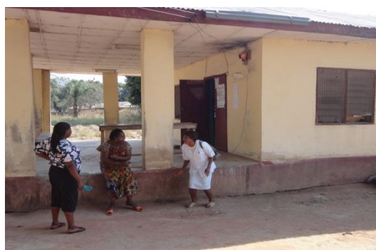
Figure 6. Front view Primary Health Care Centre Korinya (January, 2016).
