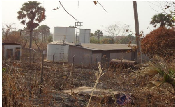
Figure 1. Abandoned Peterson Candy International (PCI) Water Works at Tse-Agberagba (February, 2016).
