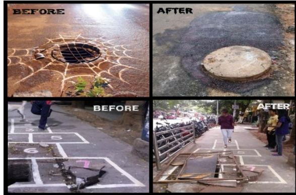
xviii. Repaired manhole after Baadal's work
