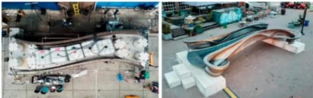
Figure 2.3 Load testing of MX3D bridge b. The MX3D bridge at Dutch Design Week [4]
